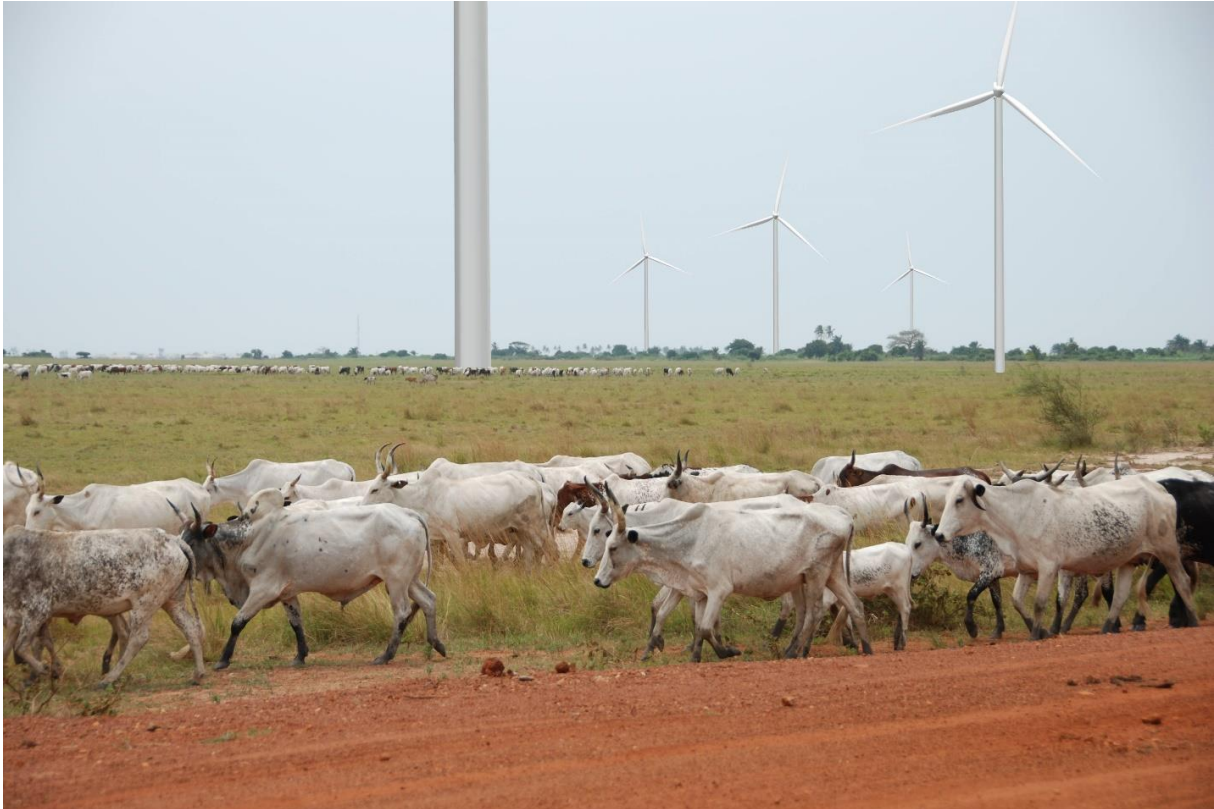
Visualization of Konikablo Wind Farm with cattle grazing in between the turbines.
