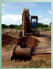
The preliminary geotechnical survey, which was already announced in previous editions of this newsletter, is completed and the relevant field work successfully carried out. The purpose of these field studies was to determine the top soil and ground structure and to obtain information on the ground water situation.
