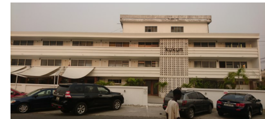
Kukun building in Accra where our new office is located.
